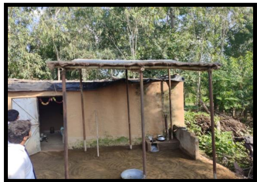
Low Cost Kitchen constructed in village Bisath.
