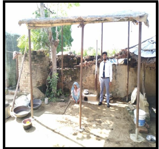
Low Cost Kitchen constructed in Trilokpuri.
