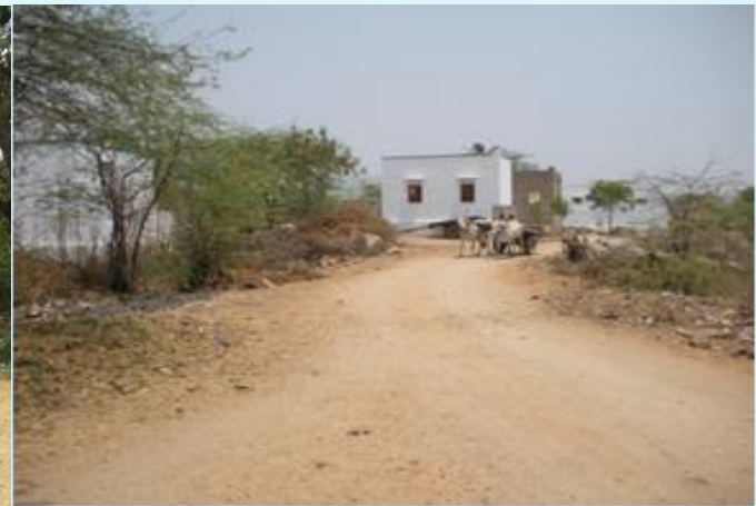
School Building and way to village from main road
