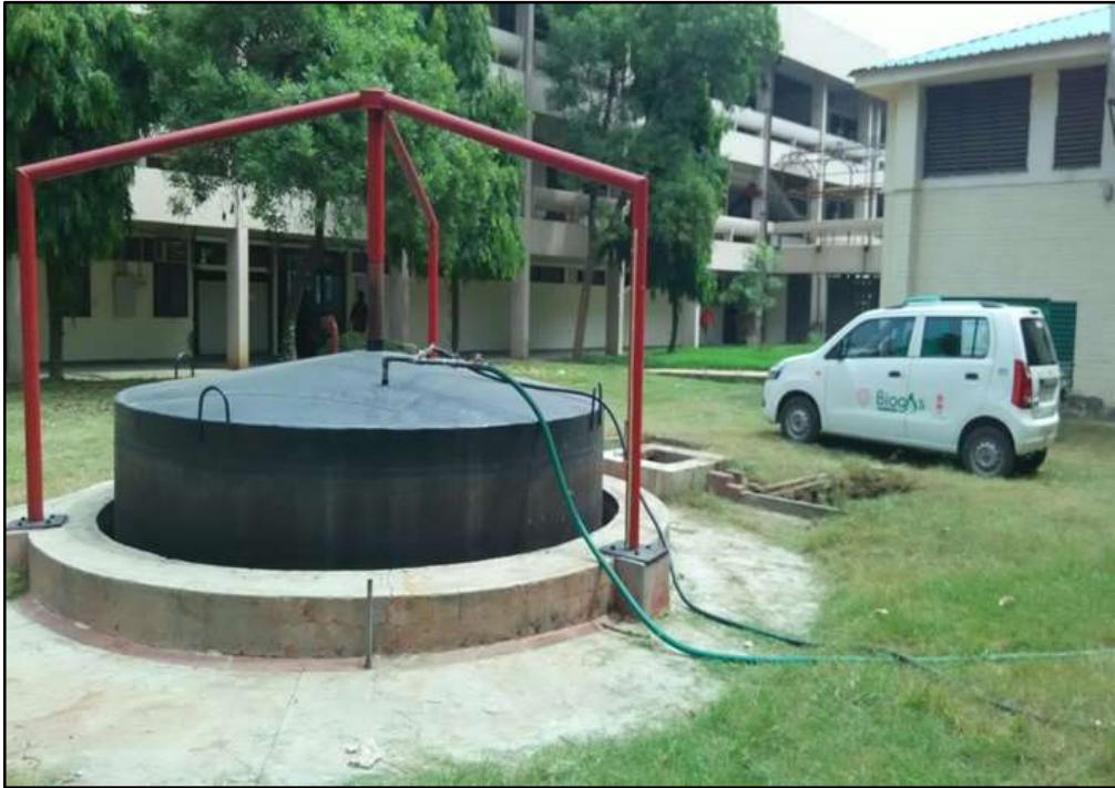
Fig. 1. KVIC model biogas plant at IIT Delhi
