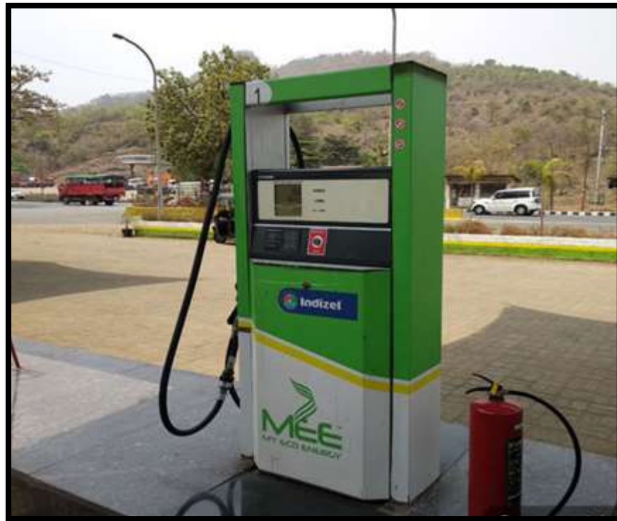
Fig. 8.4 Bio-diesel pump for fuels filling station
