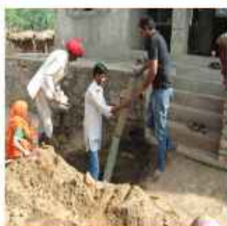
SOAK PIT CONSTRUCTION
