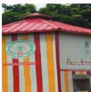
CONSTRUCTION OF P.O. PLANT IN PAMMARAKA VILLAGE
