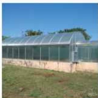
MODEL NURSERY CONSTRUCTION
