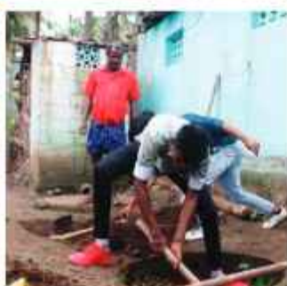
RENOVATION OF TOILETS IN PUTHUPATHE TRIBAL VILLAGE
