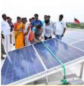
SOLAR ELECTRIFICATION STATION
