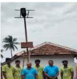
INSTALLATION OF INTEGRATED SOLAR LIGHTS
