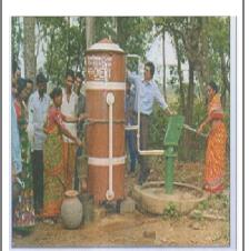
flocculation chamber and then to the sedimentation chamber. The settled water passes through plate settlers to the filter. The filtered water is drawn through tap after chlorination.
