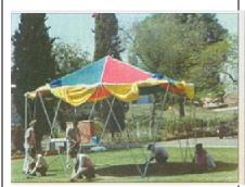
Instant shelter can be erected in 5 to 20 minutes. It is made up of triangular pipe frames joined together with the help of special joints to form a component that can be folded as one triangular bundle. Four such components having 16 triangles provide an octagonal room of 4.41 m x 4.41 m size. The cladding can be made of cloth, tarpaulin, plywood, GI sheet, thatch, insulating coverings etc. depending upon climatic conditions &resources.
