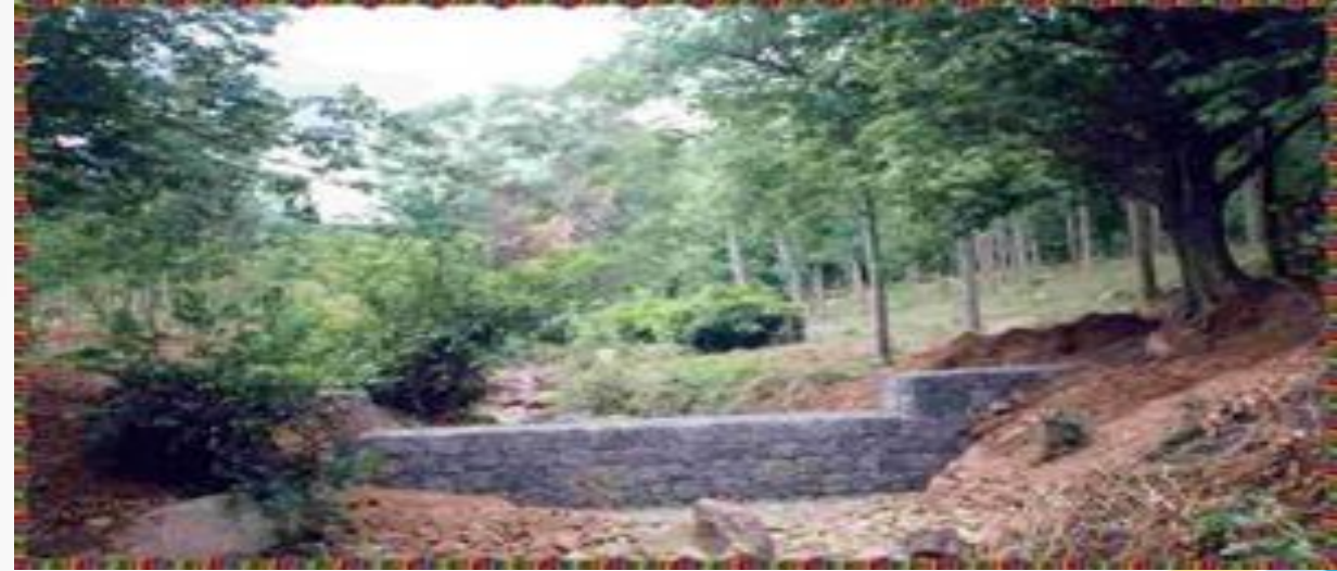
Ungated Check Dam
