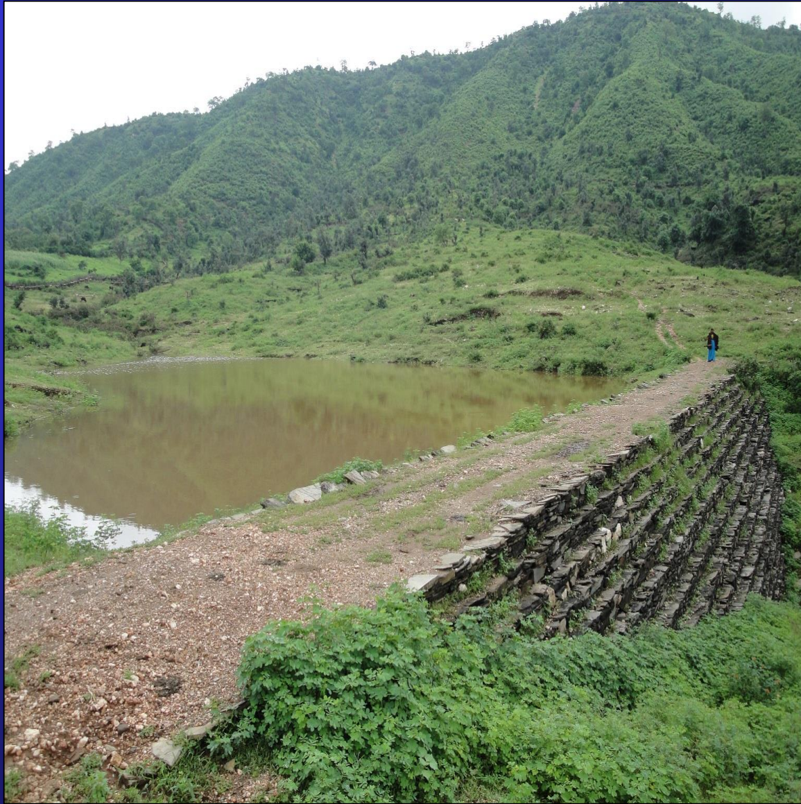
Low Cost Water Harvesting Structure
