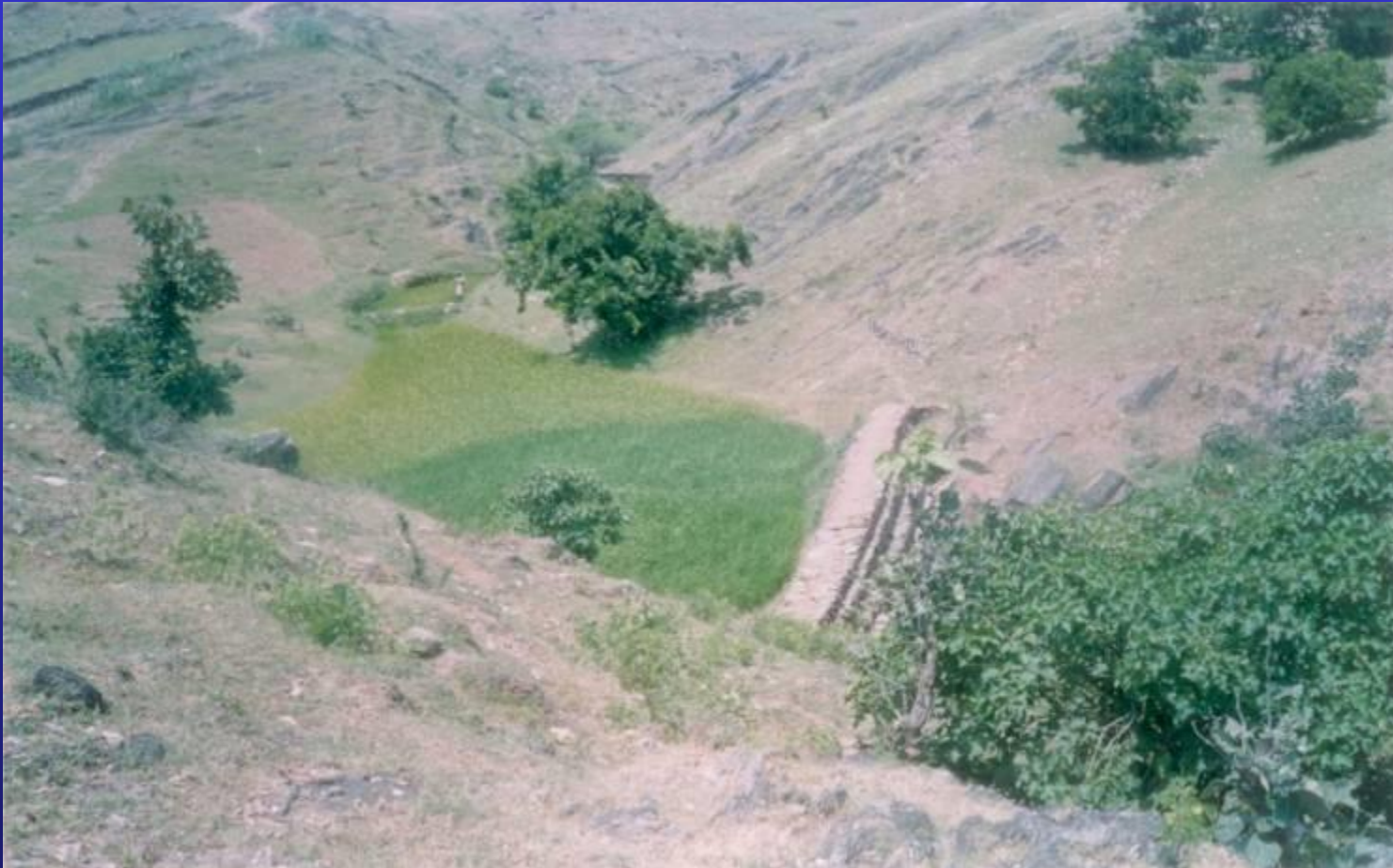
Indigenous Loose Stone Check Dam
