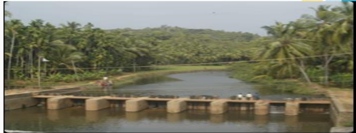
Gated Check Dam
