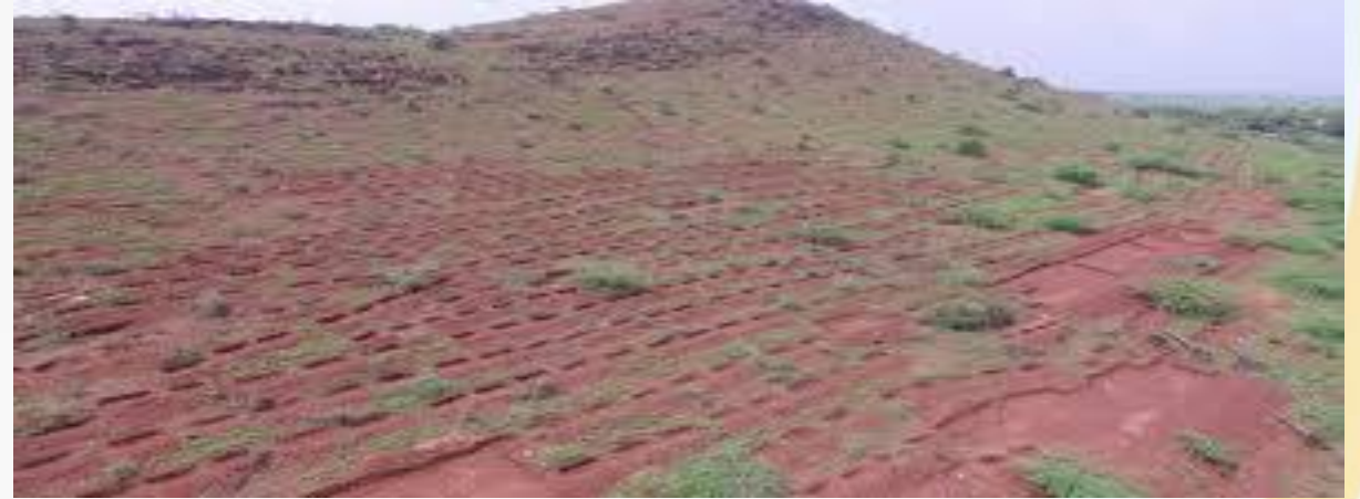
in line trenching
