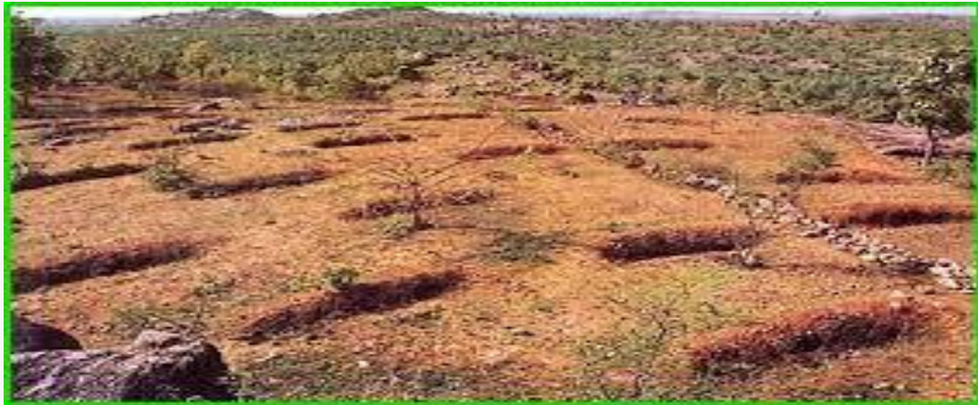
staggered trenching
