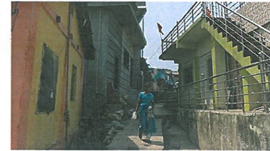
STREETS HAVE BECOME NARROW DUE TO THE UNAUTHORISED DEVELOPMENT
