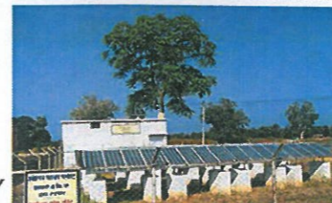
SOLAR PANELS TO INSTALLED
