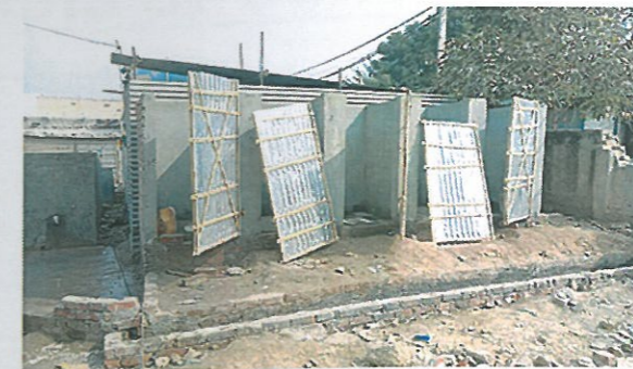
THESE ILLEGAL TOILETS ARE PROVIDING A UNHYGINIC SURROUNDING
