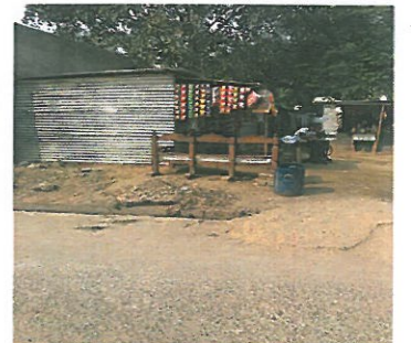
TEMPORARY HOUSES MADE OF STEEL STRUCTURES.
