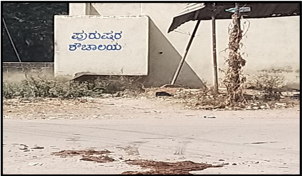
Need to built some more Community Toilet blocks
