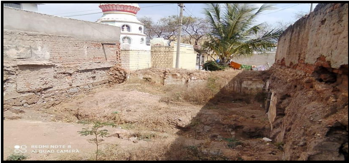
Most houses are fell due to Heavy Monsoon in Halakere Village
