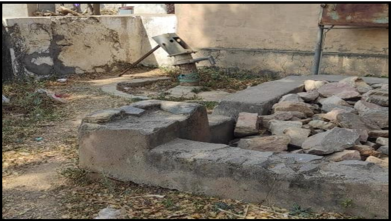
Many hand pumps are not working properly
