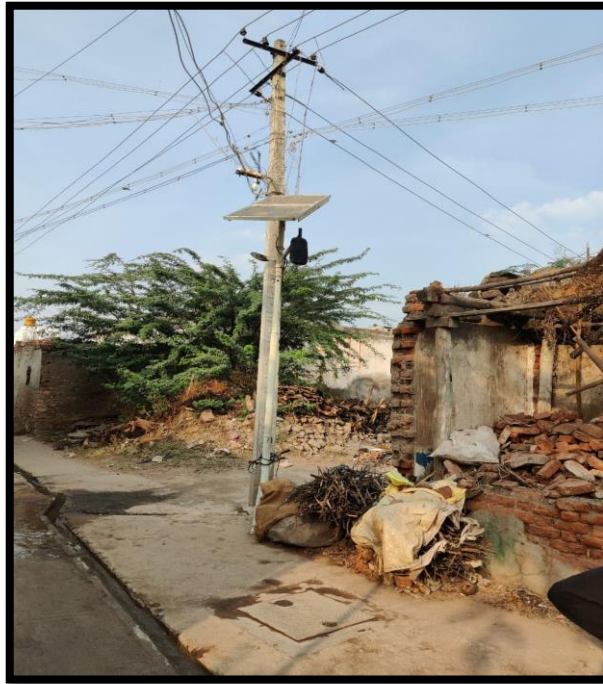
Some Houses are damaged due to heavy Rain.
