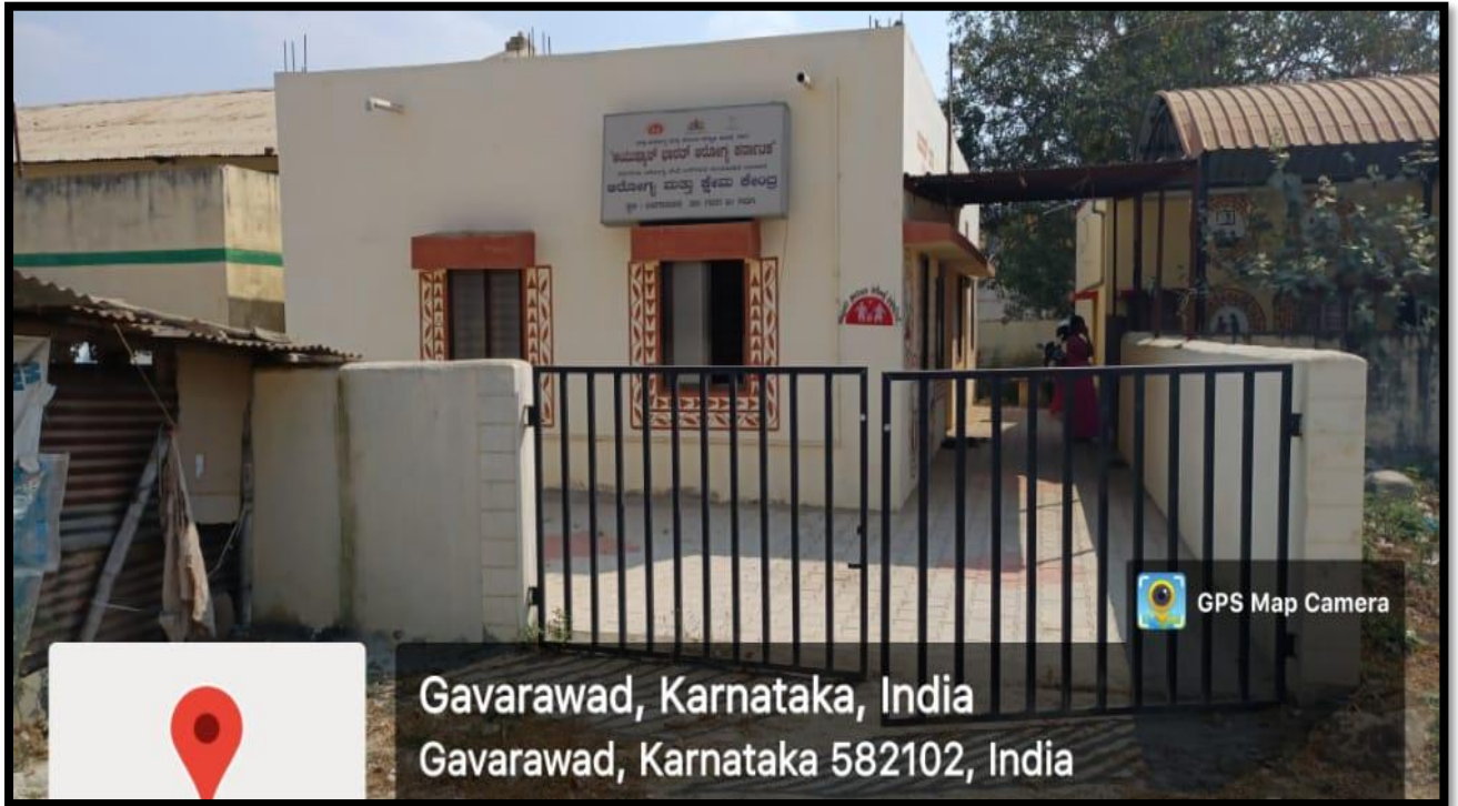
Observed Health and Wellness Centre of Balaganur Village
