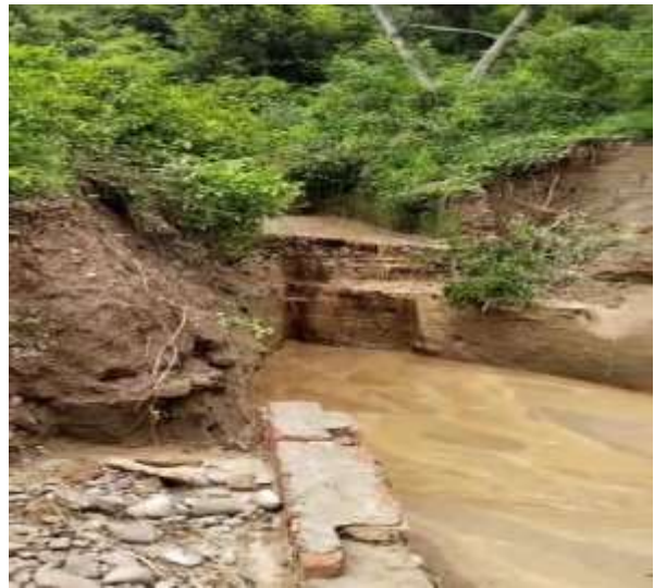
(Damaged Spillway of Majri Earthen dam due to heavy rain)
