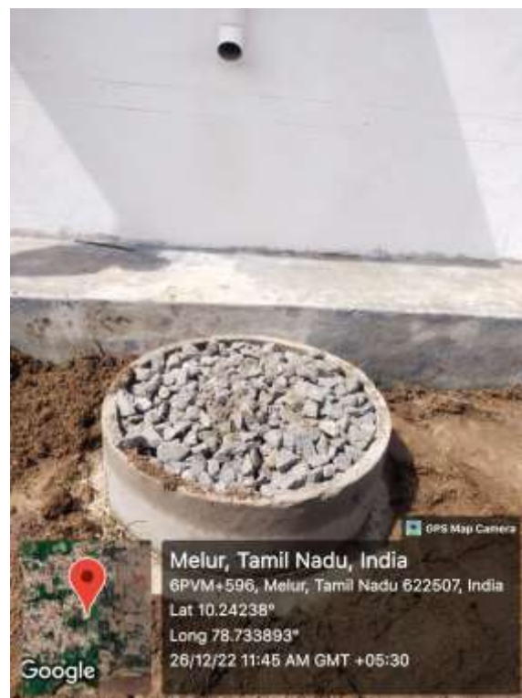
The circular rings arranged for the construction of rain water harvesting system
