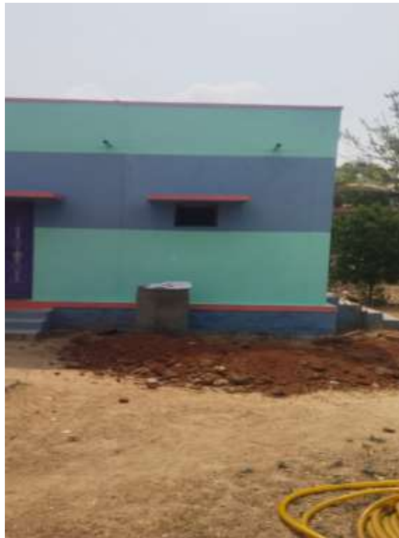
Location selected for constructing rain water harvesting system
