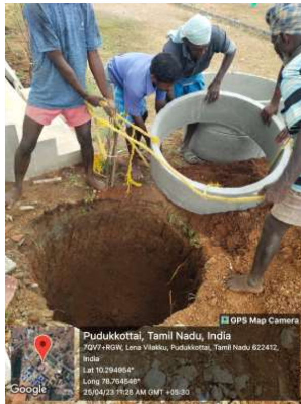
Workers placing the circular rings inside the hole with proper handling
