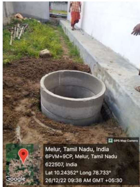
The circular rings arranged for the construction of rain water harvesting system
