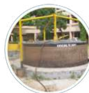
Rural Energy Systems
