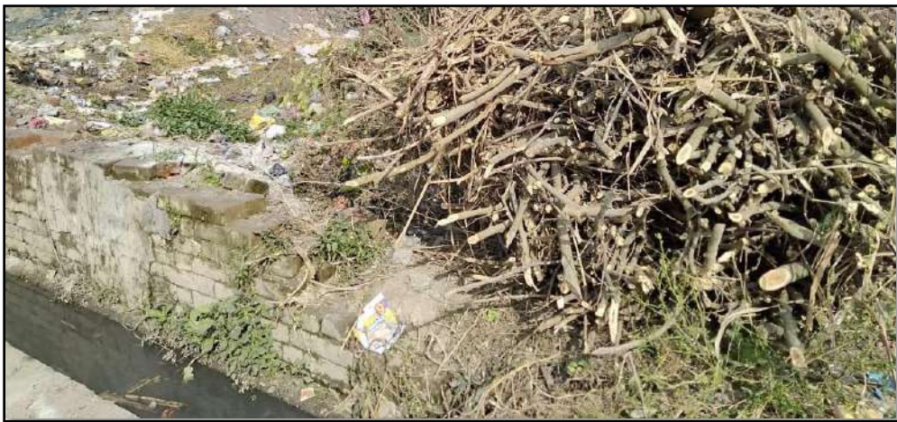
Unhygienic condition in village locality due to dumping of solid waste and flowing of contaminated water
