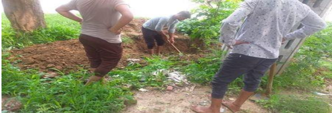
b. picture after complete digging
