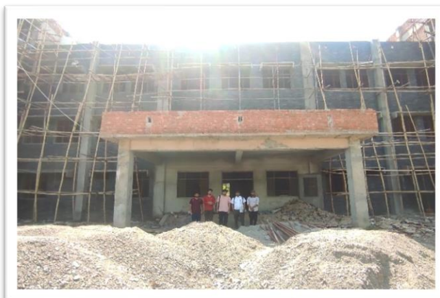
Model Degree College (Under Construction)
