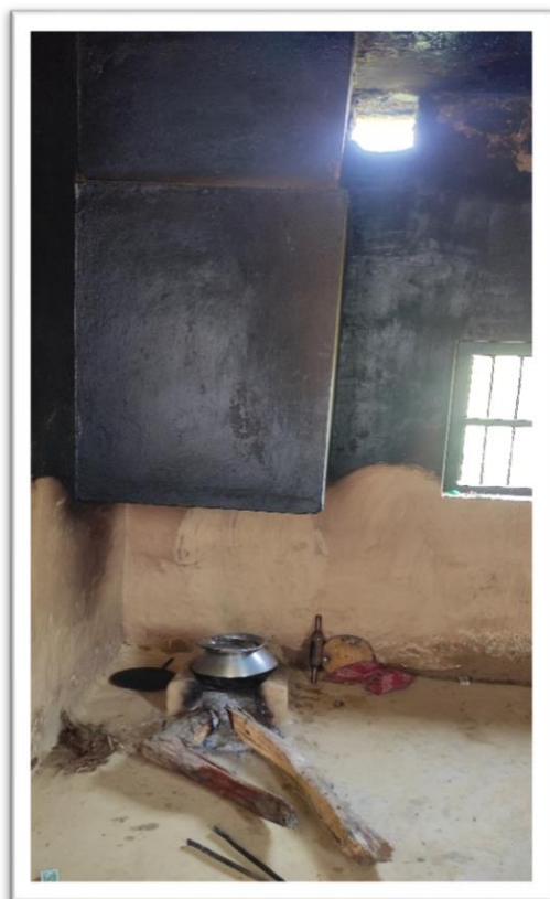
Inefficient chimney design in the kitchen, Peeli Padav
