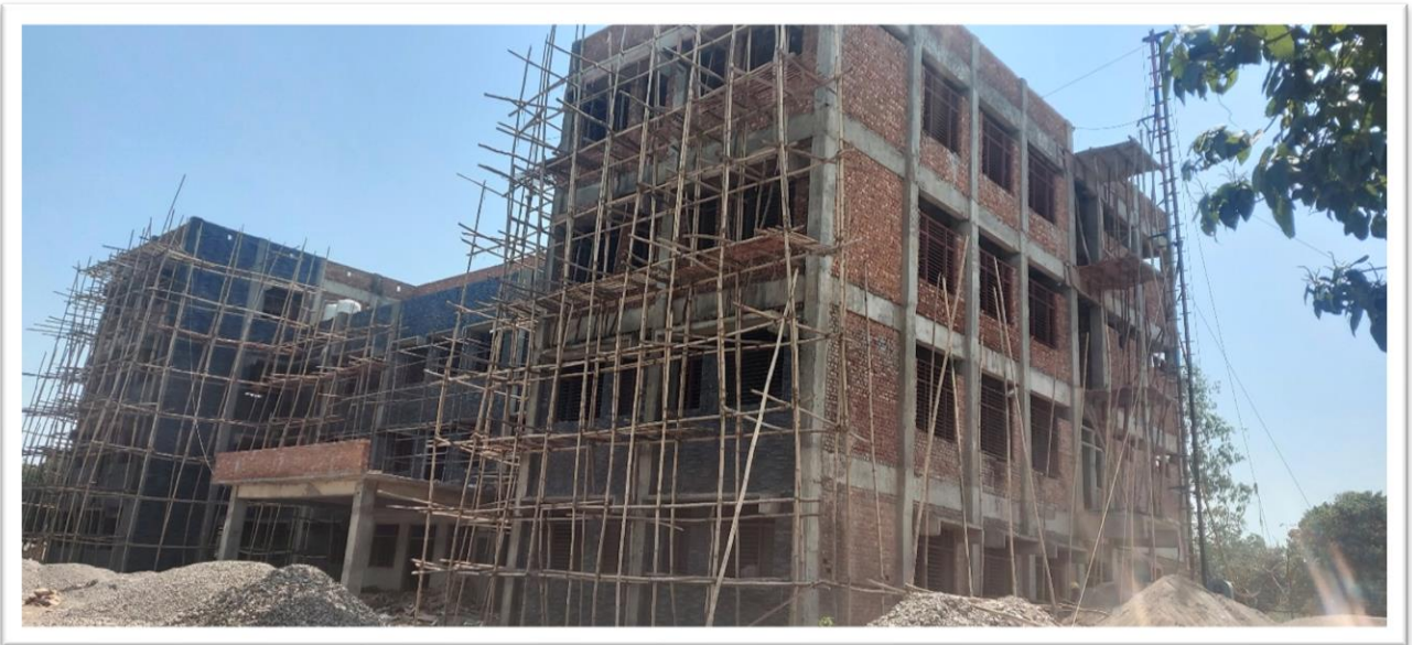
Current status of ongoing construction of model degree college
