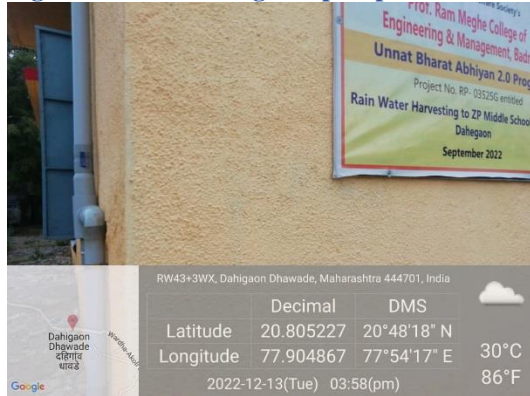
Figure 6: RWH filter installed and UBA banner
