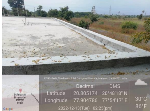
Figure 5: Slab flooring and parapet work completed
